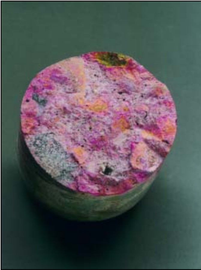
Concrete Core Showing Advanced ASR
